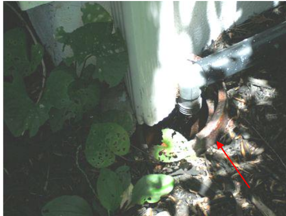
Old underground clay pipe
