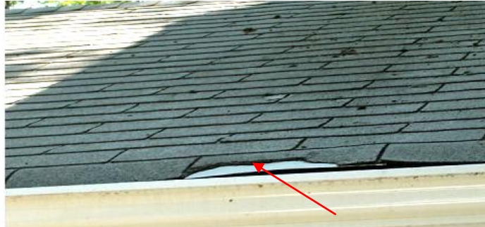
The Roof is Worn – example of broken shingle shown here
