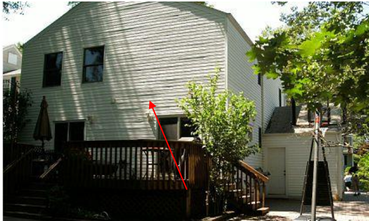
Vinyl Siding Shows Irregular Surface
