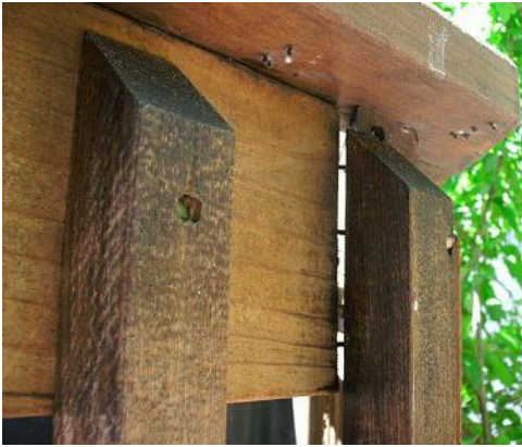
Separation in deck railing
