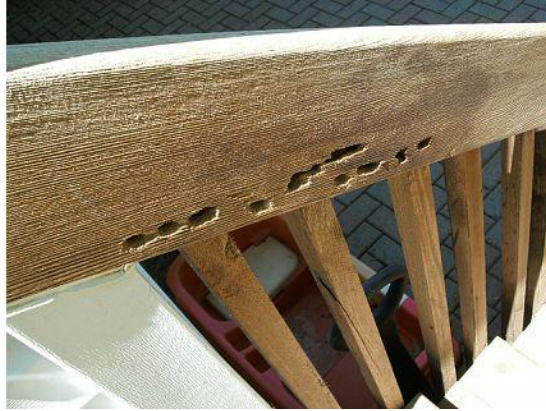
Carpenter bee damage
