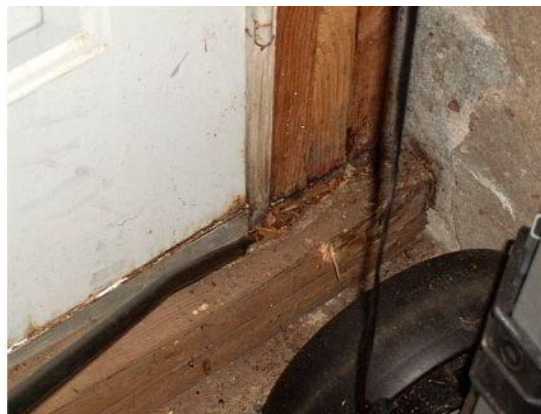
Carpenter ant damage section of the sill plate
